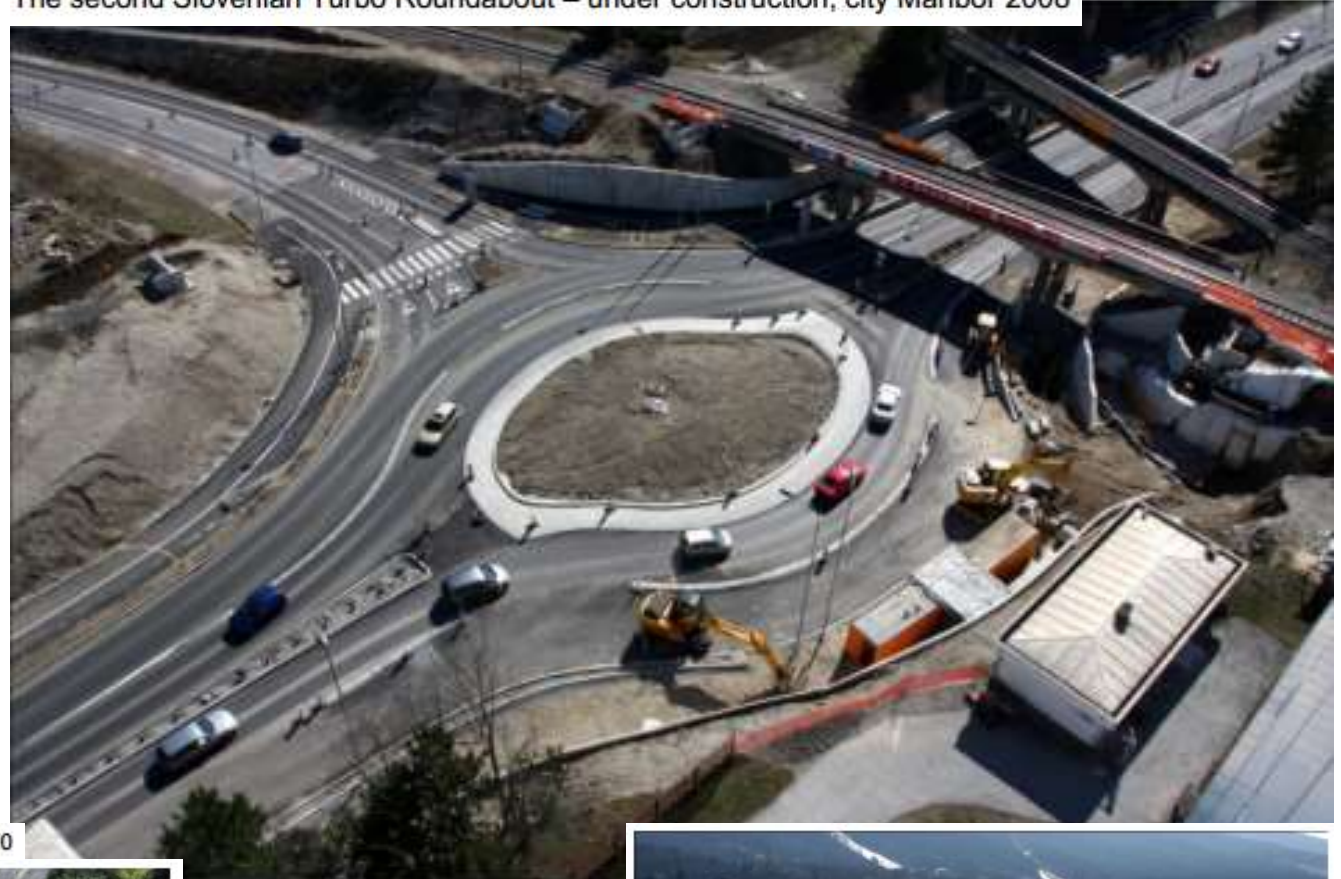
The second Slovenian Turbo Roundabout – under construction; city Maribor 2008
